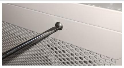
**NOTE:** Safety cables will be attached to the diffuser face, but care should be taken to ensure that diffuser face does not swing and injure anyone.
