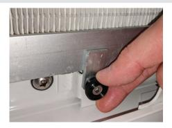
STEP 3: Turn all cam latch filter retainers to the open position.
