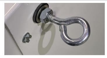
Step 6: Adjust and level the unit so that it rests on the tees and there is adequate compression on the gasket to warrant a tight seal.
